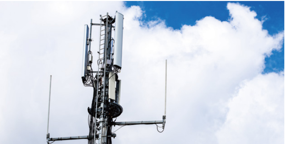
China Tower Heilongjiang Smart Sodium Battery Project
