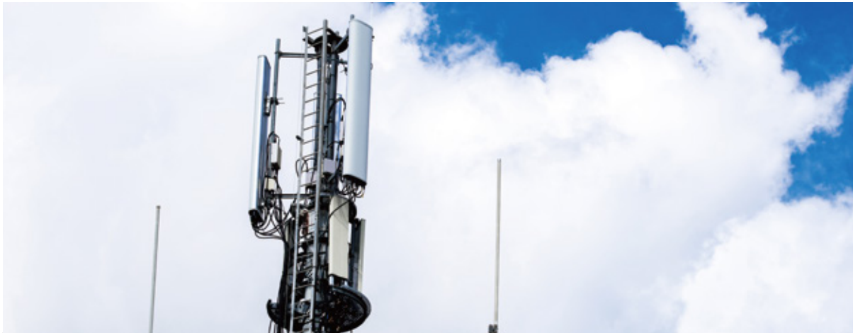
China Tower Heilongjiang Smart Sodium Battery Project
