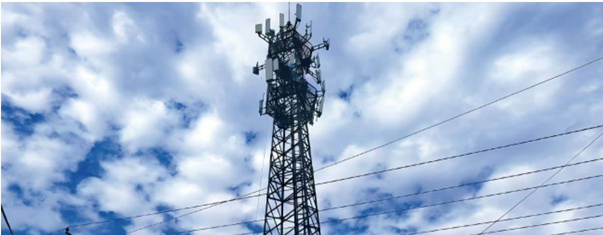
China Mobile Heilongjiang Smart Sodium Battery Project
