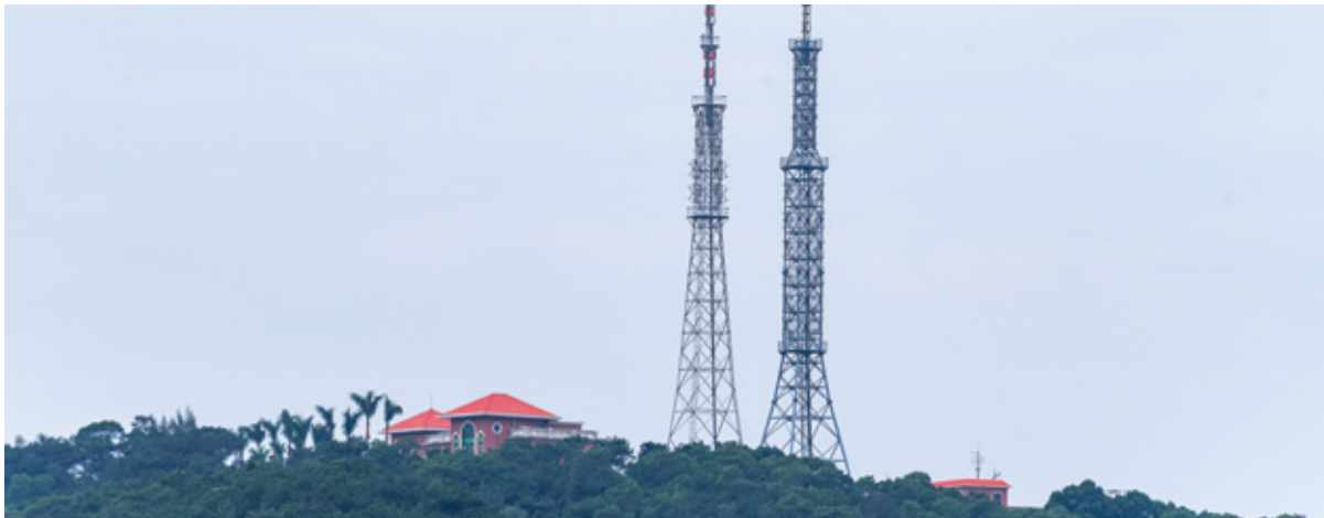
Cambodia Metfone Base Station Project
