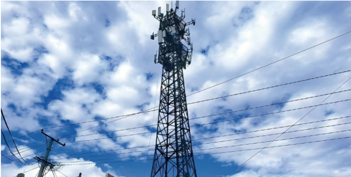
China Mobile Heilongjiang Smart Sodium Battery Project Project Time: 2024 Project Location: Heihe,Heilongjiang, China
