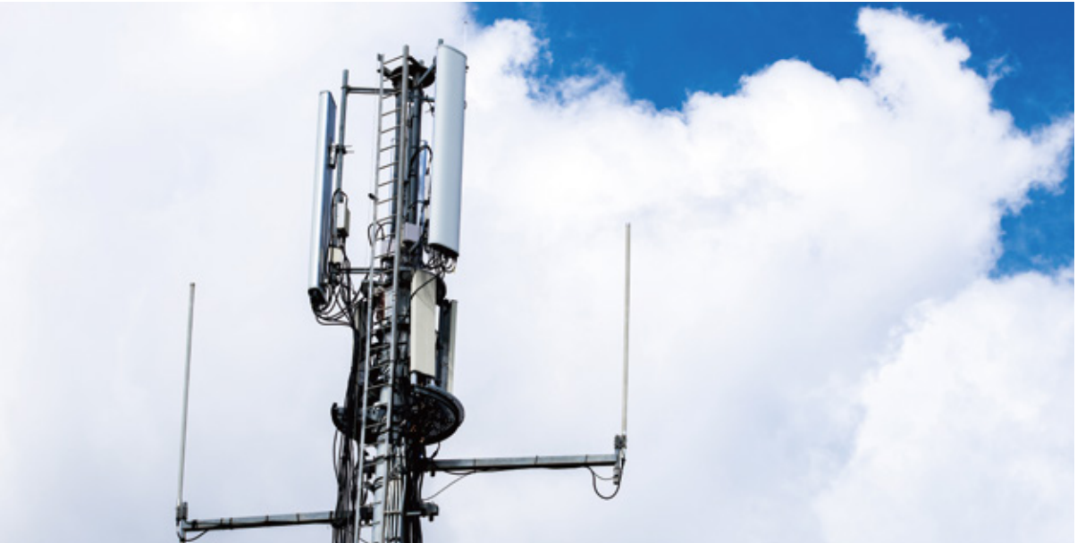
China Tower Heilongjiang Smart Sodium Battery Project Project Time: 2024 Project Location: Qitaihe,Heilongjiang, China
