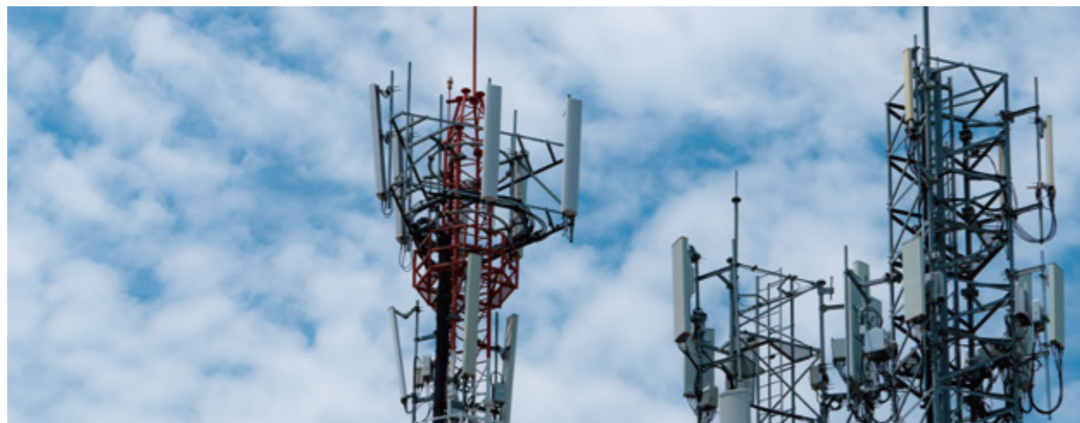
China Mobile Hunan 5G Micro-Station Integrated Project
