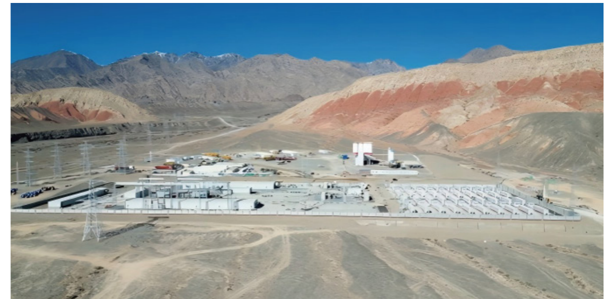
Xinjiang Wuqia 50MW Wind Power + 50MW/200MWh Energy Storage Project
