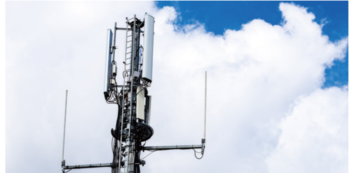
China Tower Heilongjiang Smart Sodium Battery Project
