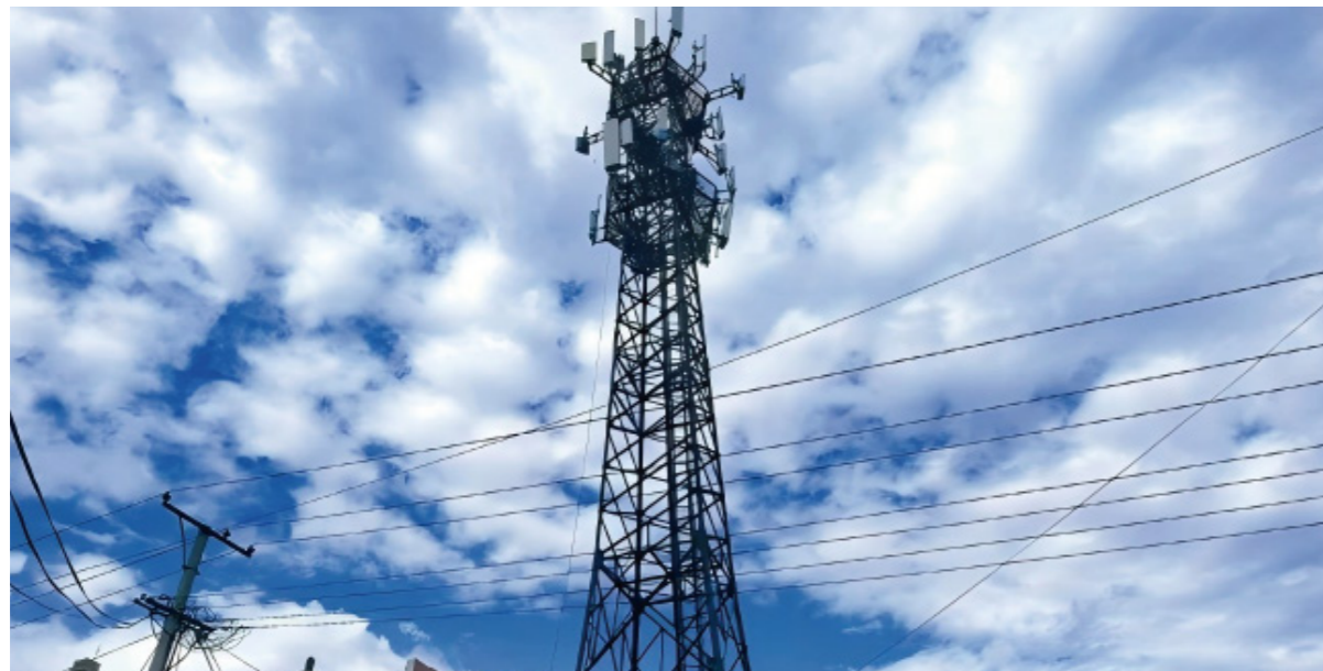
China Mobile Heilongjiang Smart Sodium Battery Project
