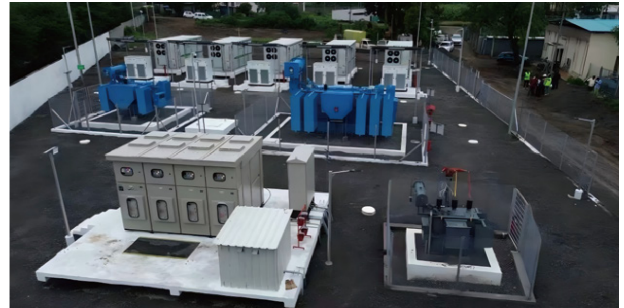
India 11MW/22.99MWh Energy Storage Project Project Time: 2025 Project Location: India Project Highlights: Wind power paired with energy storage to smooth output.
