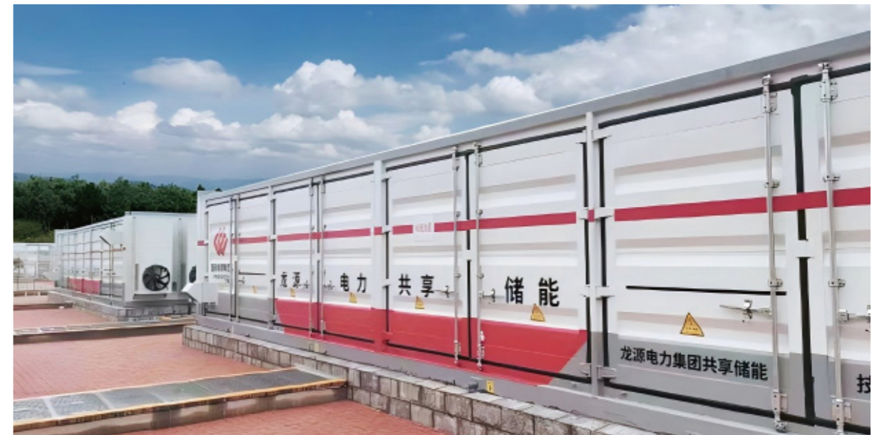
Guizhou Weining 80MW/160MWh Wind Power Energy Storage Project
