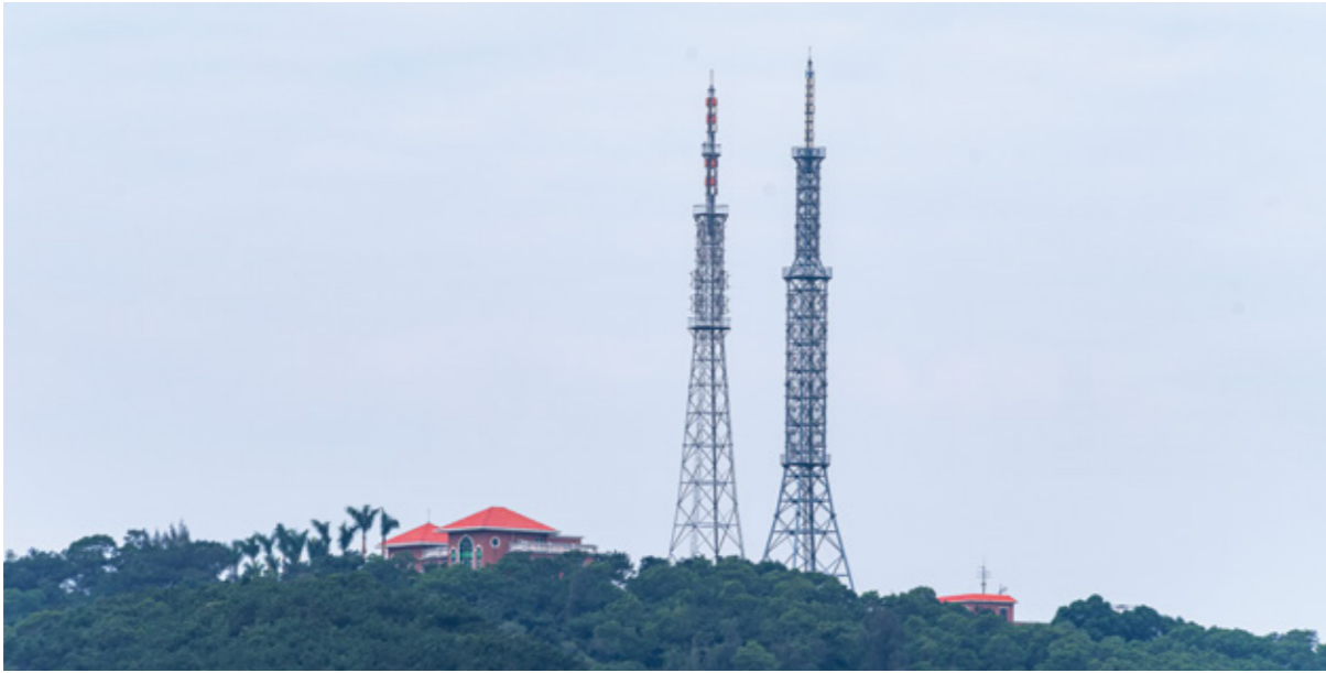
Cambodia Metfone Base Station Project
