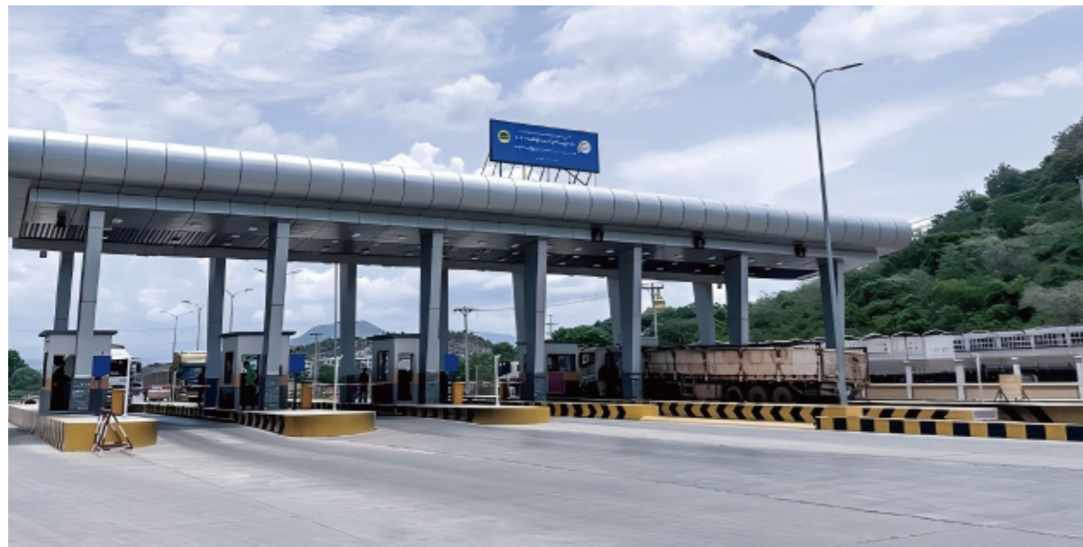
Myanmar Mandalay SKG Toll Station Commercial & Industrial Energy Storage Project
