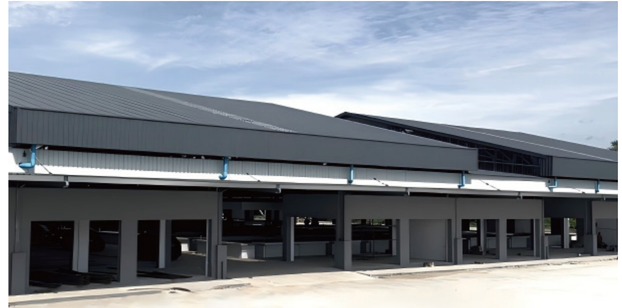
Myanmar Mandalay Farmers' Market Commercial & Industrial Energy Storage Project
