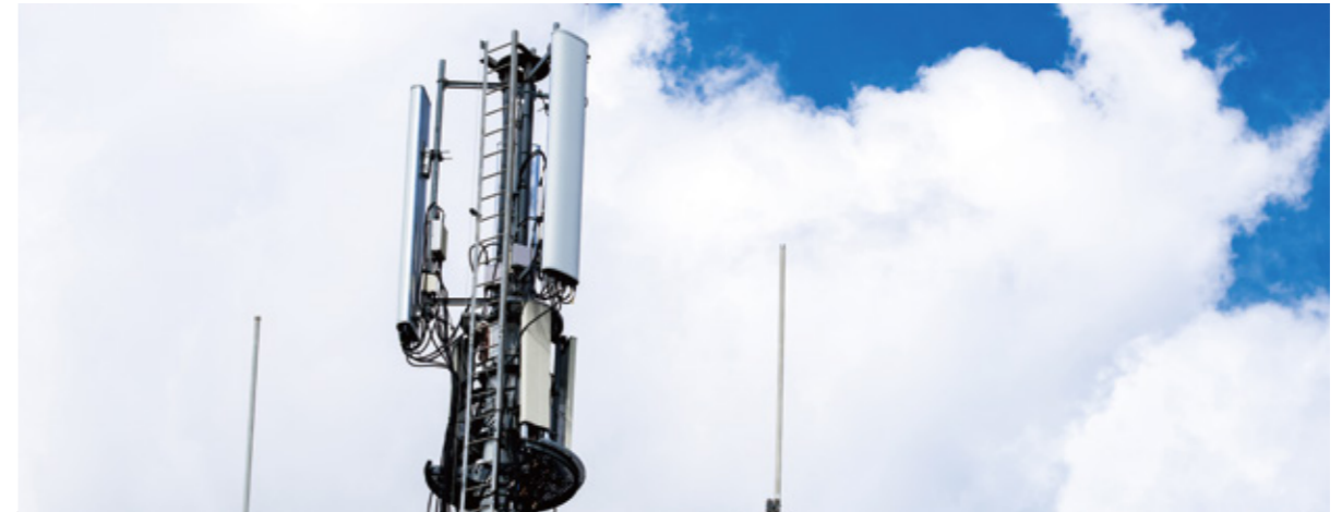
China Tower Heilongjiang Smart Sodium Battery Project
