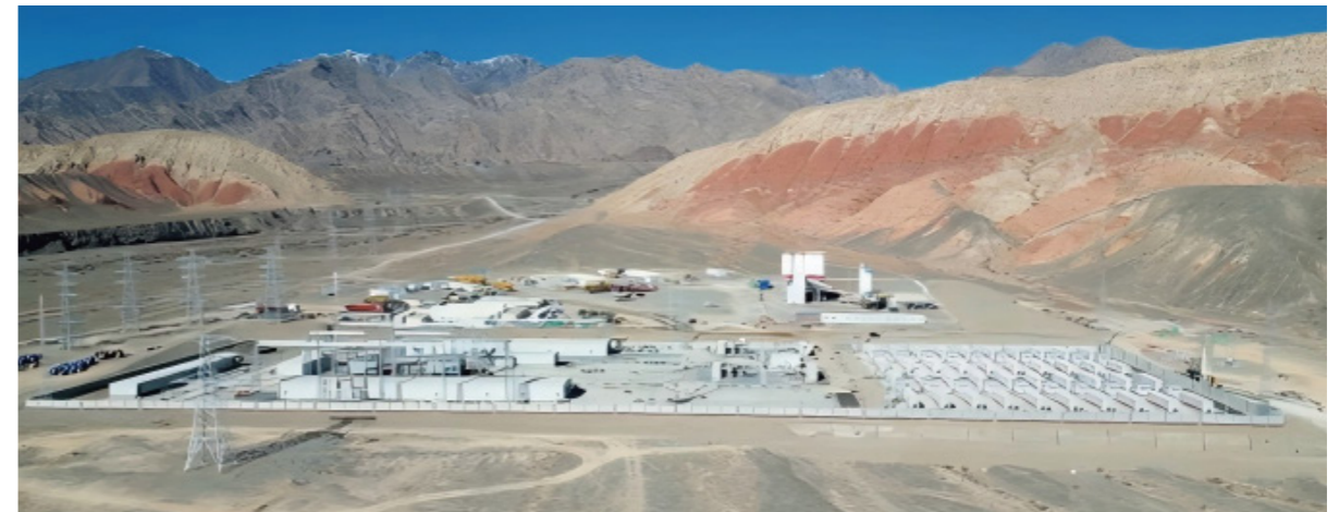
50MW Wind Power Generation and 50MW/200MWh Energy Storage Project in Wuqia, Xinjiang
