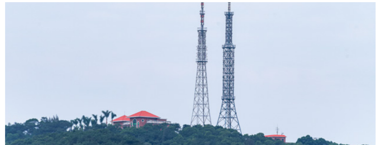
Cambodia Metfone Base Station Project
