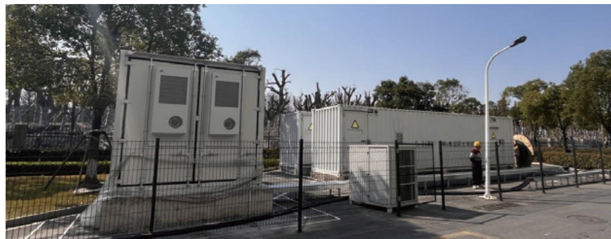
Shanghai Mobile Lingang IDC Data Center UPS Project
